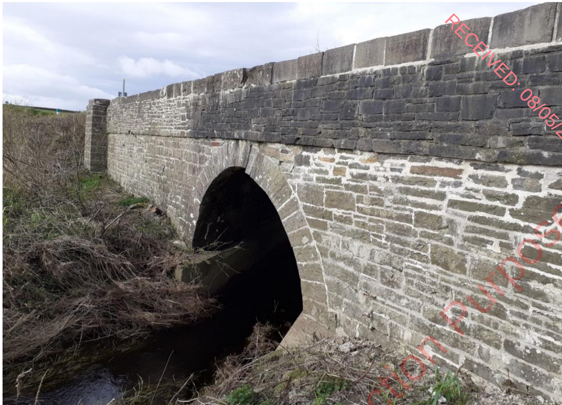
Plate 4.3. Option 2 GCR runs along the R483 for a short stretch and passes over Cavanagh's Bridge, which is a substantial stone arch structure (April 2023).
