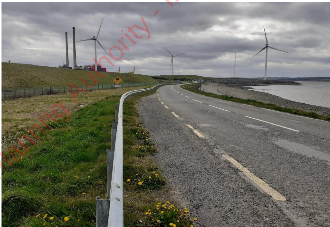
Plate 4.6. Option 2 GCR runs along the N67 leading towards the Moneypoint facility for approximately 500 m. The road is above the shoreline, with grassy verges along both sides. Looking southeast (April 2023).
